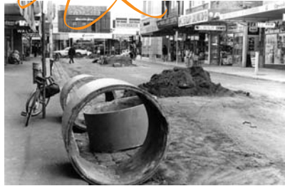
Eaton Street 1978 – during construction of Mall (Photo: The Oakleigh Historical Society)
