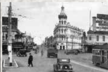
St Kilda Junction St Kilda Melbourne, 1930s
