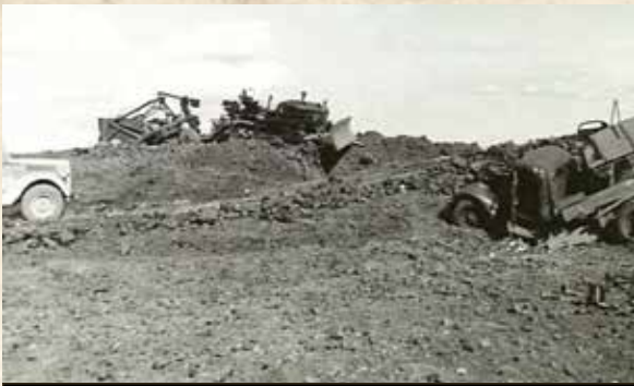
The approach to Farsala bridge from the north, after German aircraft had scored a direct hit on a truck loaded with ammunition. Farsala, 18 April 1941. Photo S B Cann. AWM
